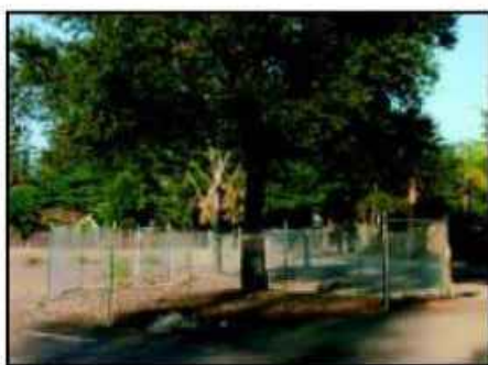
IMAGE 2.15-2 Tree Protection Fence at the Dripline
