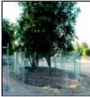
IMAGE 2.15-1 Tree Protection Fence at the Dripline
