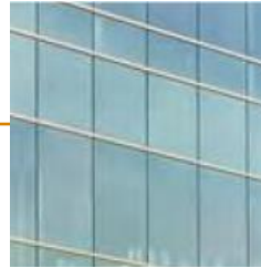
GL-1 BUTT-JOINT CURTAIN WALL GLAZING
