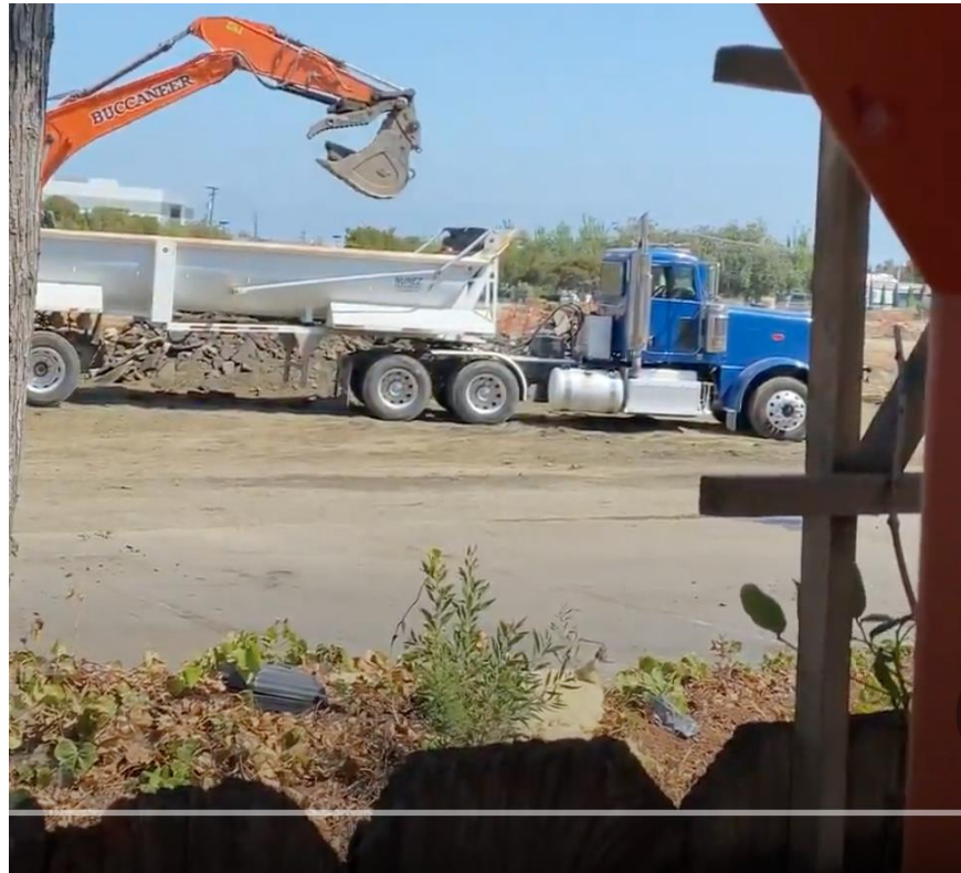
Image 3: Improper use of loaders and hauling trucks, with excess drop height, new residences.
