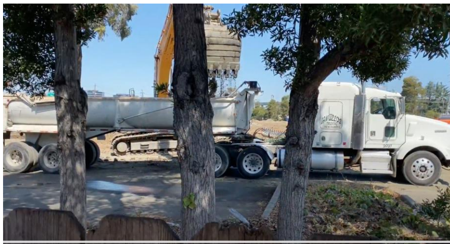
Image 4: Improper use of loaders and hauling trucks, with excess drop height, new residences.
