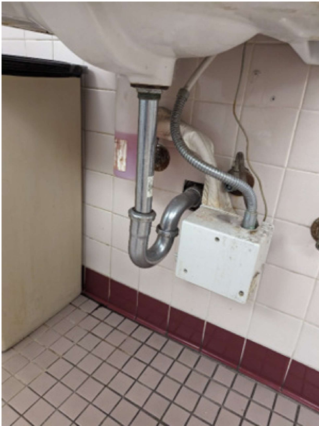
Undercounter Electric Tankless Water Heaters
