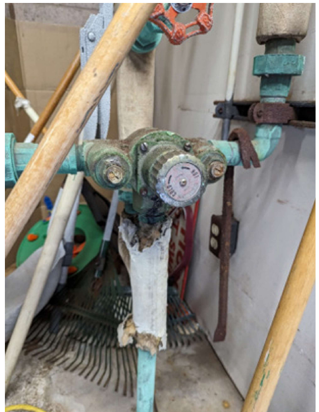
Central Thermostatic Mixing Valve beside the tank
