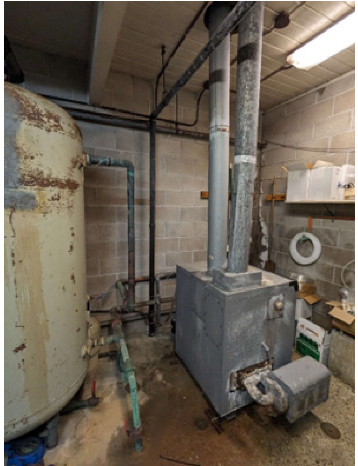
Gas Fired Water Heater and Tank
